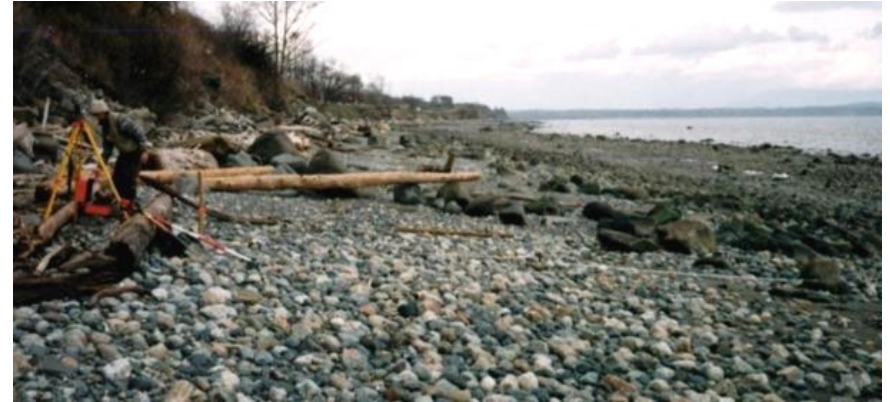
Lummi Shore Road Before/ After revetment and nourishment
