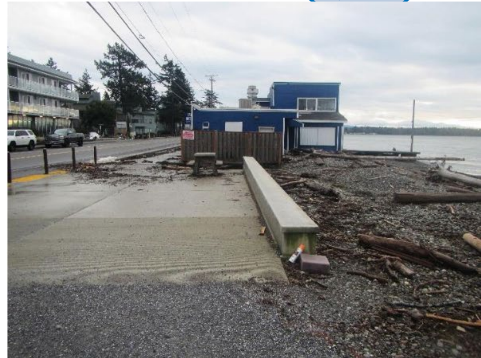
High water debris line near 31+00, Jan 2022.
