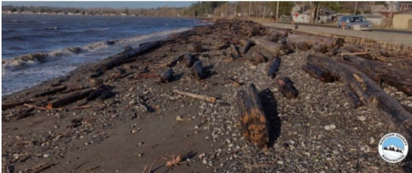
BERM AND RESTORED NATURAL SHORELINE AFTER JAN. 13, 2021 STORM SHOWING LOGS PUSHED UP BEACH, BUT NOT ON THE ROADWAY.
