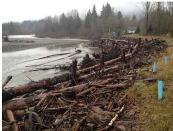
**Fig. 6** ELJ installed as large wood revetment for bank protection along South Fork Nooksack River, Whatcom County, WA. *Reference Module in Earth Systems and Environmental Sciences, (2018)*
