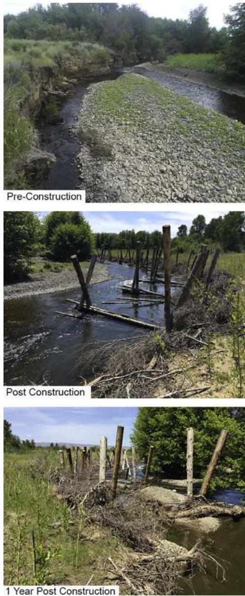
**Fig. 8** ELJs installed in Toppenish Creek in 2016 to raise bed level, water levels and stabilize high banks lacking riparian trees. Yakima County, WA.
