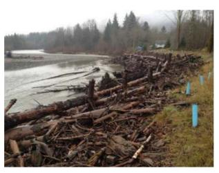
Fig. 6 ELJ installed as large wood revetment for bank protection along South Fork Nooksack River, Whatcom County, WA.
