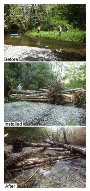
Fig. 14 Pre- and postproject conditions and 1-year post project conditions for ELJ retaining sediment in Big Beef Creek, Kitsap County, WA. View looking downstream.
