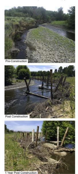
Fig. 8 ELJs installed in Toppenish Creek in 2016 to raise bed level, water levels and stabilize high banks lacking riparian trees. Yakima County, WA.
