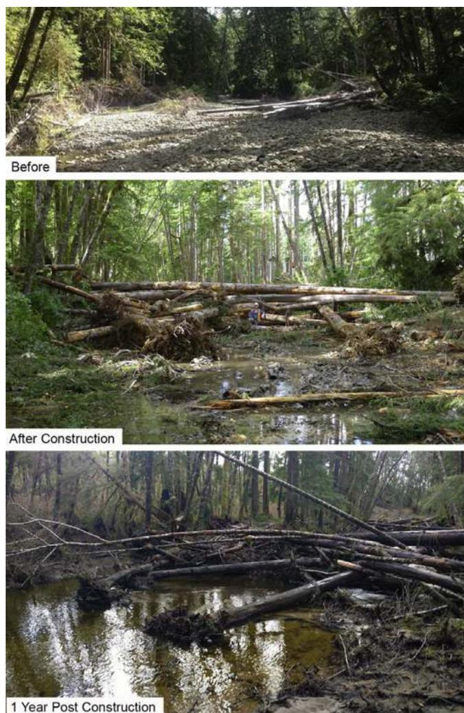
**Fig. 19** Valley scale ELJ, pre-construction, post construction and 1 year afterwards. Hurst Creek, Jefferson County, WA.
