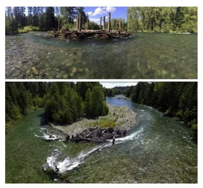
Fig. 17 Two examples of apex ELJs, Cle Elum River, Kittitas County, WA.
