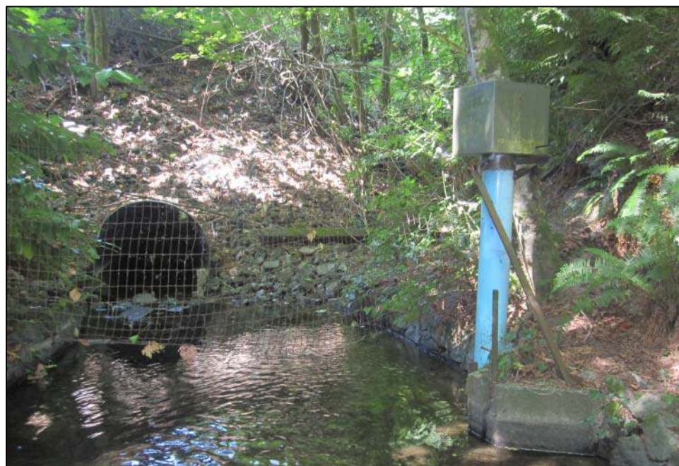
Figure 59. Photo of partial barrier to fish passage in Kitsap Creek at Northlake Way NW (view downstream). Photo taken August 2012 by Steve Todd, Suquamish Tribe.
