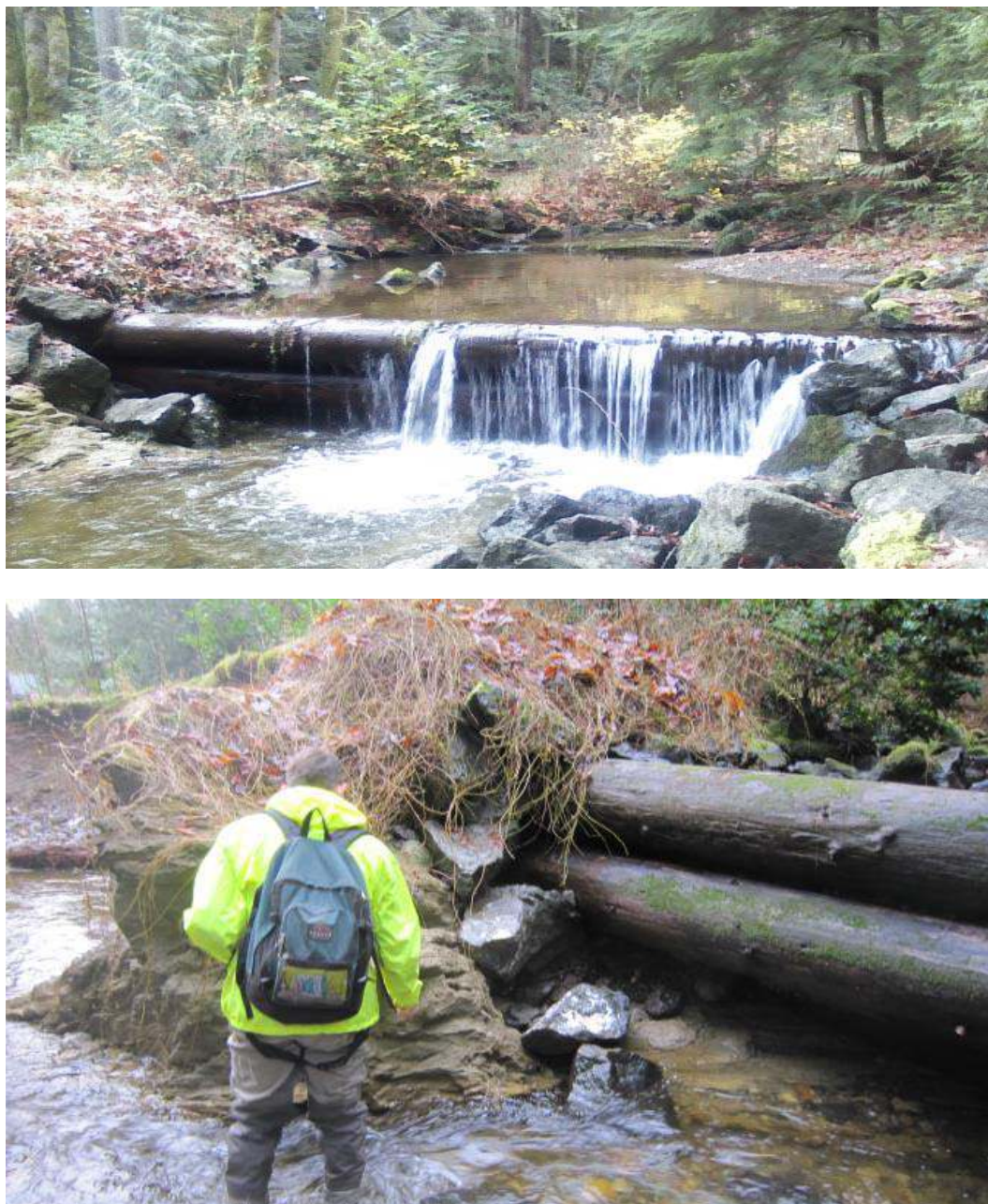
Figure 62. Photos of log weirs on Dickerson Creek downstream of Navy railroad in 2007 (Upper; photo by Jon Oleyar, Suquamish Tribe) and in February 2013 (Lower; photo by Paul Dorn, Suquamish Tribe). Note erosion around failing weir in 2013.
