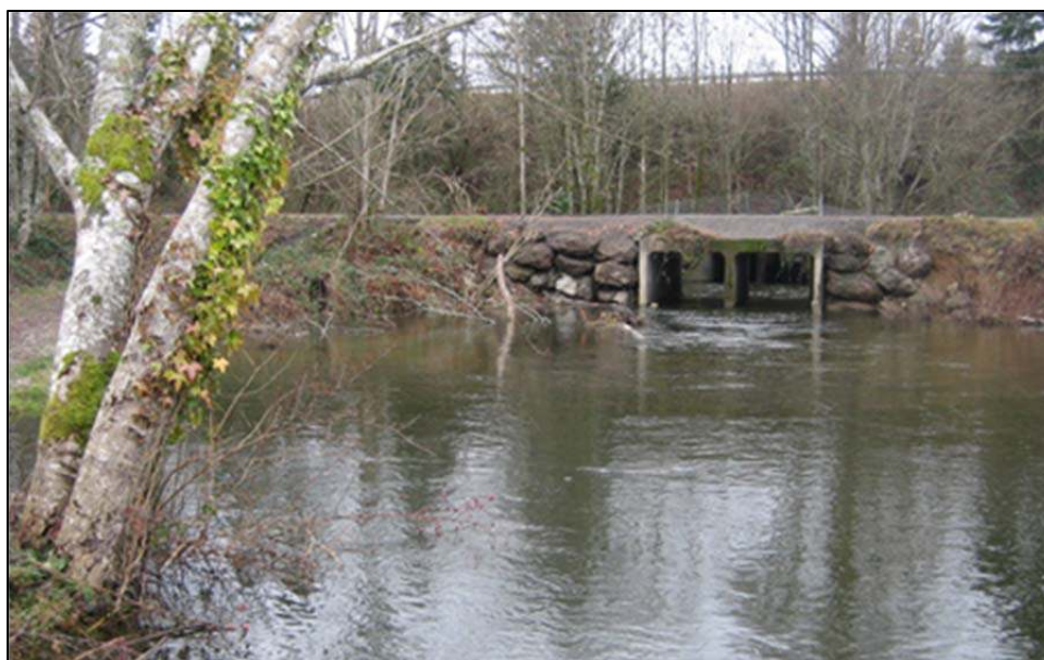
Figure 46. Photo of double box culvert at Kittyhawk Drive (view upstream). Photo taken from Habitat Work Schedule, credit unknown.
