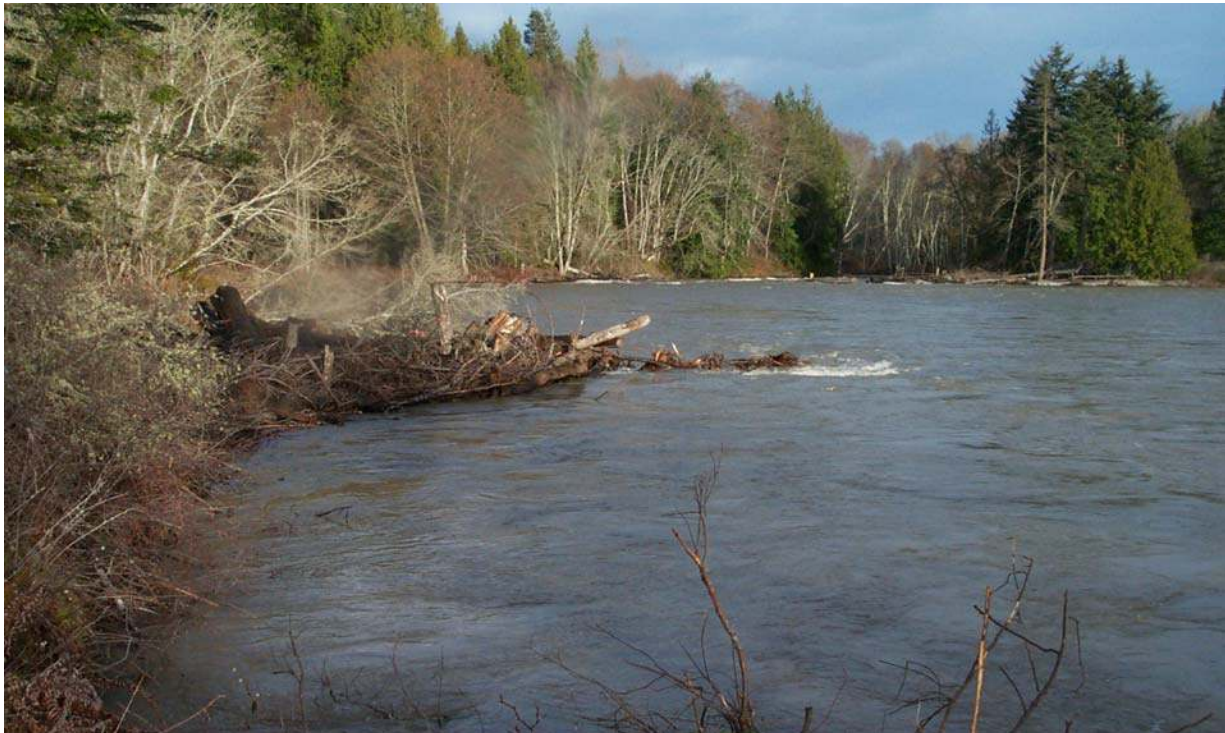
Figure 47. Elwha River engineered logjam #99-3, winter 2002. Photo taken from left bank looking North (downstream) at inlet to HRC.
