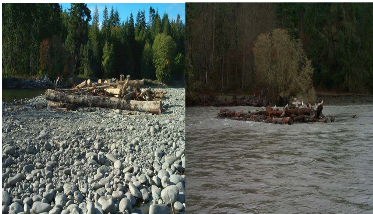
Figure 38. Elwha engineered logjam 02-2 immediately following construction in 2002 (left) and at typical winter discharge. Photos are looking Northwest in the direction of flow.
