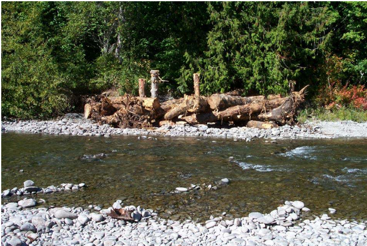
Figure 43. Elwha engineered logjam #02-3 located on left bank of EMC, immediately following construction, September 2003. Photo taken from right bank looking North across EMC.
