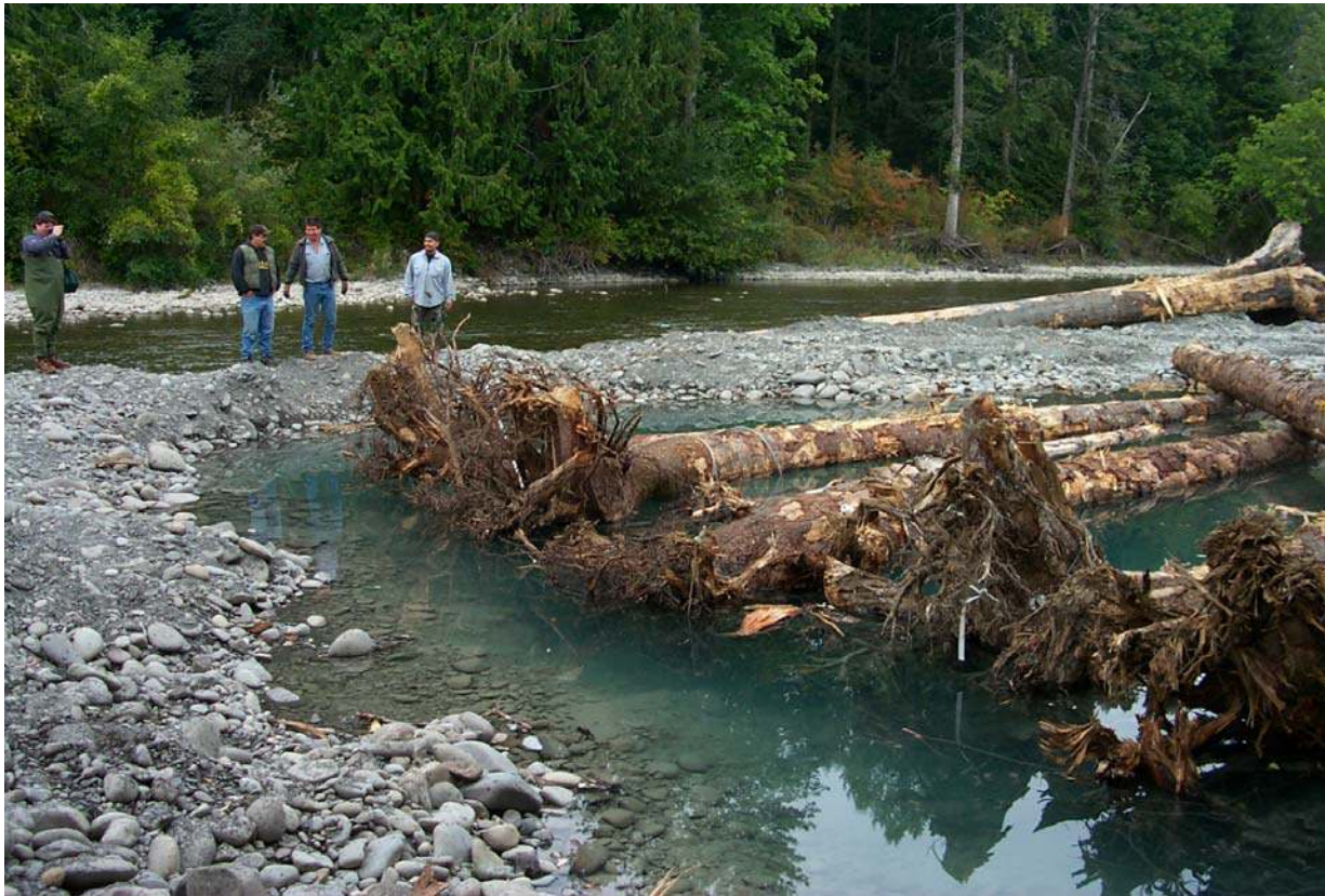
Figure 42. Elwha engineered logjam #01-1 during construction, August 2001. Photo from right bank looking North across the EMC.
