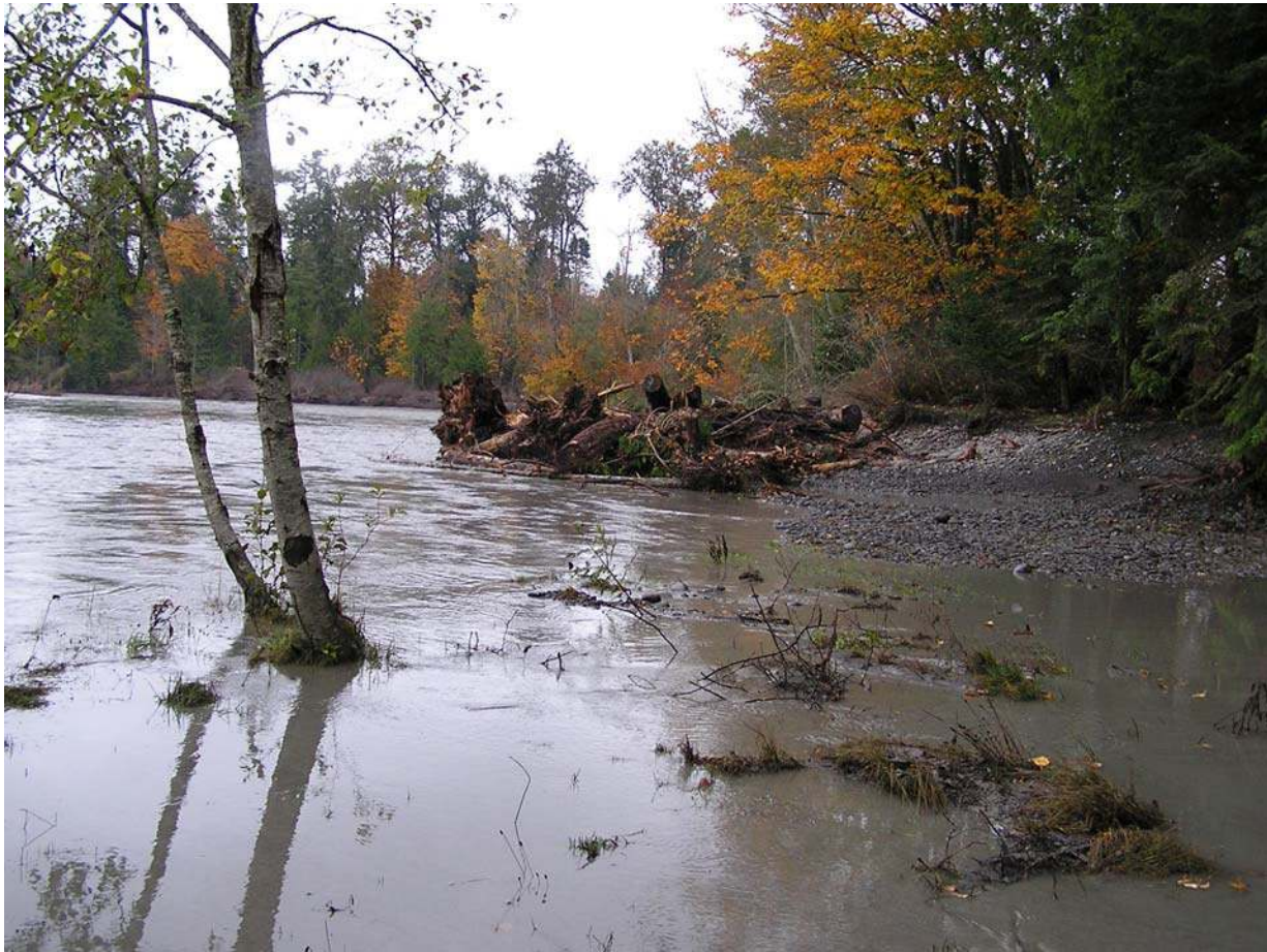
Figure 45. Elwha engineered logjam #03-2, winter 2004. Photo taken from right bank looking North (downstream).
