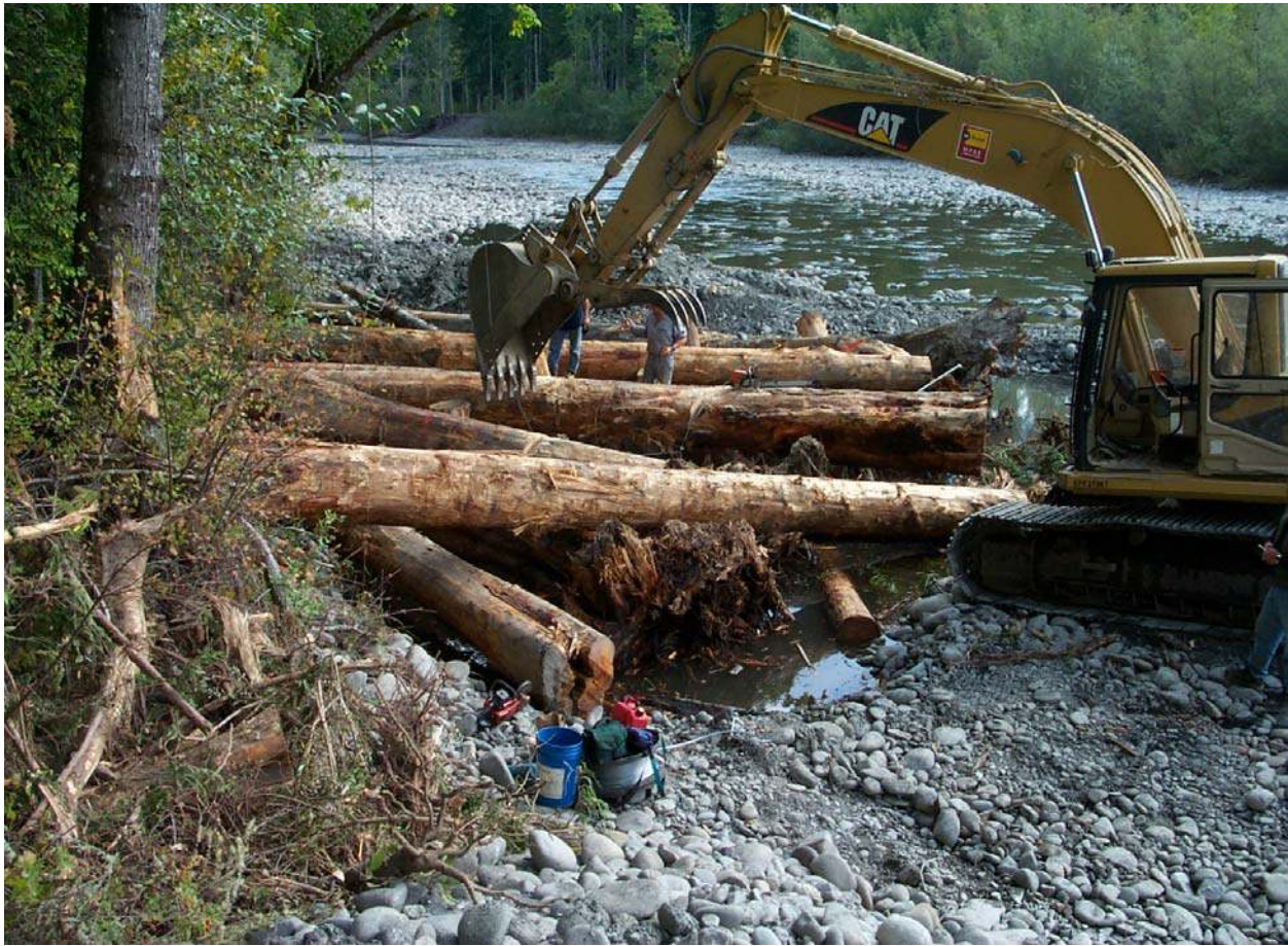
Figure 41. Elwha engineered logjam #01-3 during construction, August 2001. Photo taken from the left bank looking East-Northeast (downstream).
