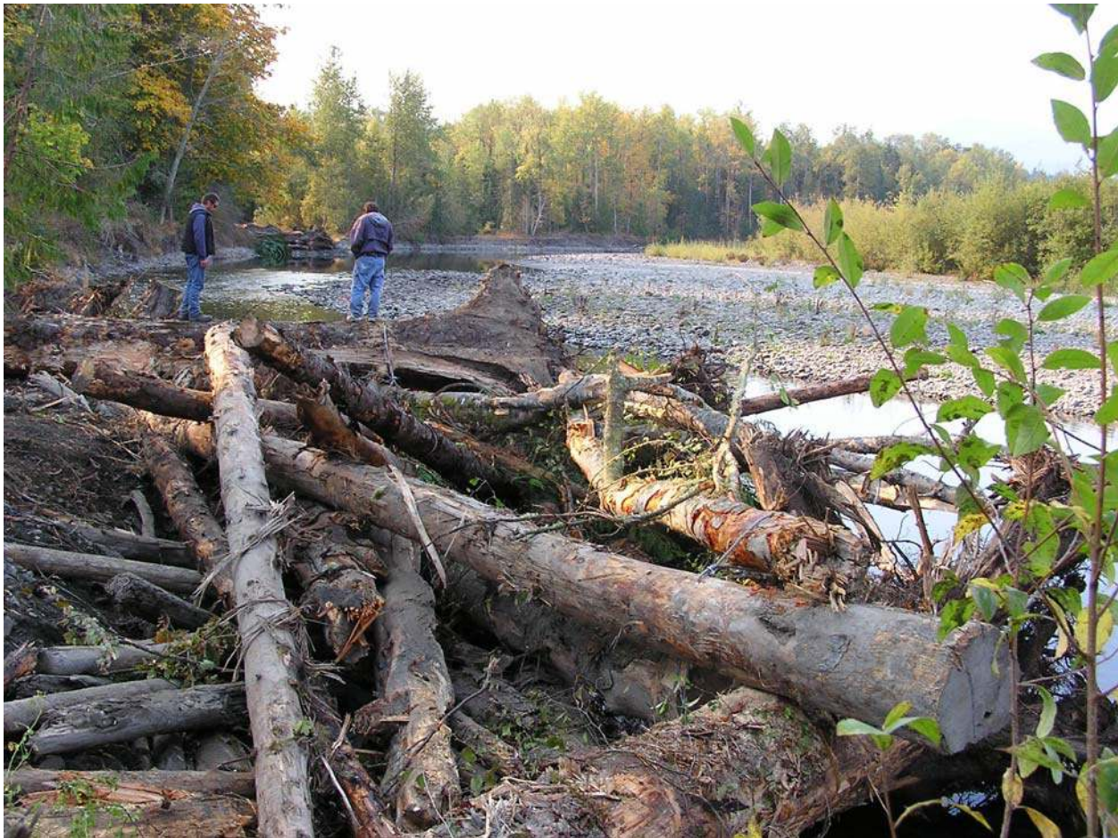
Figure 44. Elwha engineered logjam #03-1 immediately following construction, August 2003. Photo taken from right bank of EMC looking South (upstream). ELJ 03-2 is visible in background (left center of photo).
