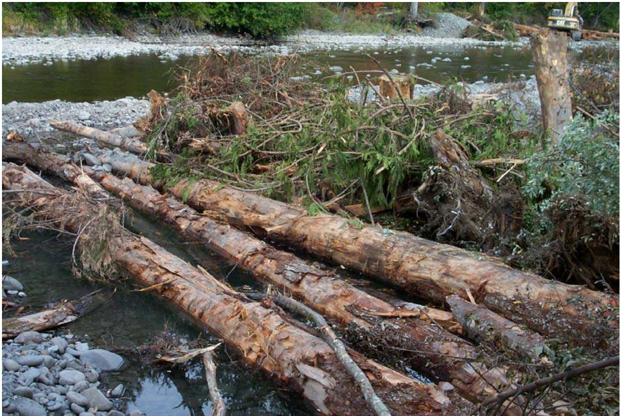
Figure 36. Elwha engineered logjam #01-1 immediately after completion, fall 2000.
