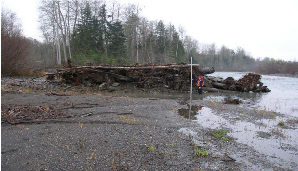
Figure 52. Elwha engineered logjam #04-2 situated along the left bank of the EMC immediately downstream of where a HRC distributary channel re-enters the EMC (visible on left), winter 2007. Photo taken from left bank of EMC looking North (downstream).
