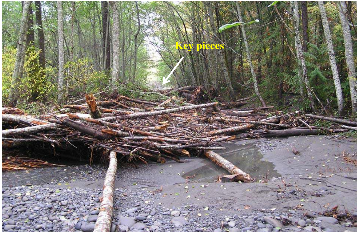
Figure 53. Logjam formation upstream of 2003 unanchored key pieces placed in Side Channel 5. Photo taken after October 2004 flood flow, looking Northeast (downstream). Alder trees visible in photo are racked up on key pieces and were eroded from upstream floodplain as Side Channel 5 increased in size due to flood flows. The side channel is almost devoid of wood upstream of this location. ELJ 00-1 is located at inlet to Side Channel 5 and may have contributed to the increase in flow down the side channel.
