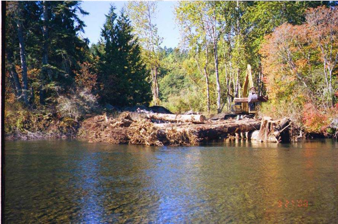
Figure 48. Elwha River engineered logjam #00-2 located along left bank of Sisson property, during construction, fall 2000. Photo is taken from gravel bar looking West across the river.
