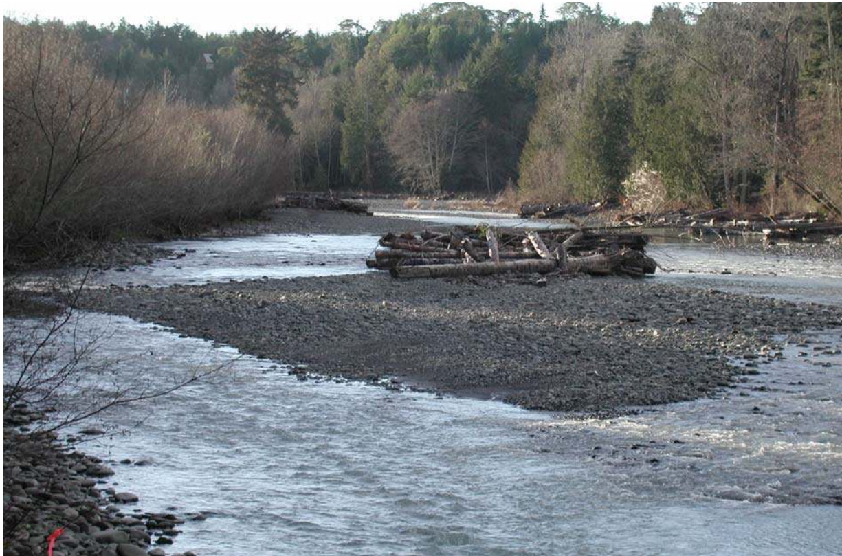
Figure 40. Elwha engineered logjam #02-5, December 2005, three years after construction. Note large gravel bar behind structure. Photo is looking West-Southwest up the EMC from the right bank.
