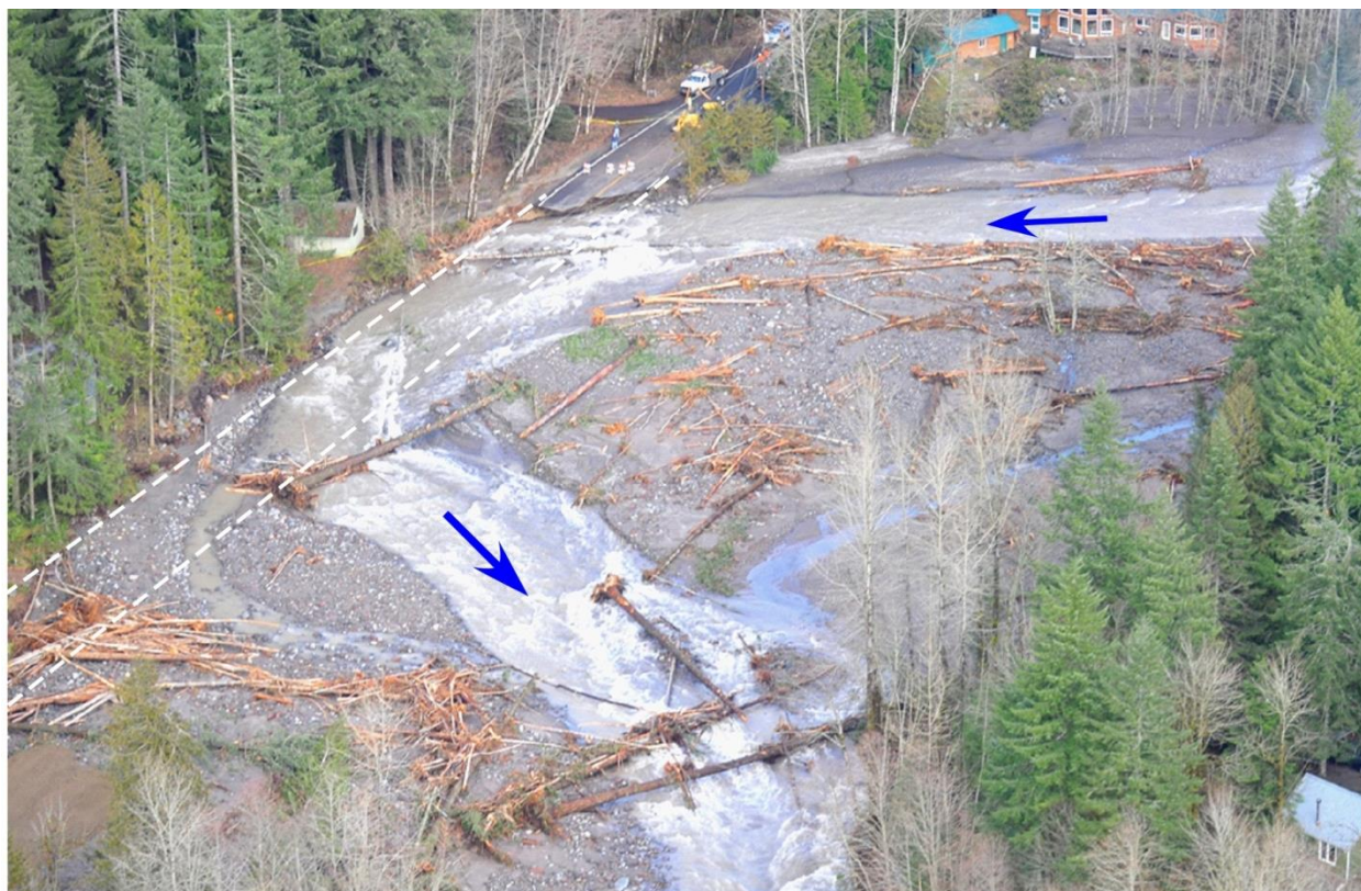
Figure 32. Upper Sandy RM 44.1 Lolo Pass Road washout in 2011. The channel moved through the road adding over 60 ft to its migration zone. The flood left a net increase in the quantity of wood in the channel which added additional flow resistance and enhanced fish habitat. Historic confinement and wood clearing has concentrated the river's energy and severely limited the formation of beneficial salmon habitat. Providing the river with more room to move and implementing flood protection measures that focus on energy dissipation will not only improve habitat but reduce long-term flood protection costs. In this case the road was rebuilt in its pre-existing location.
