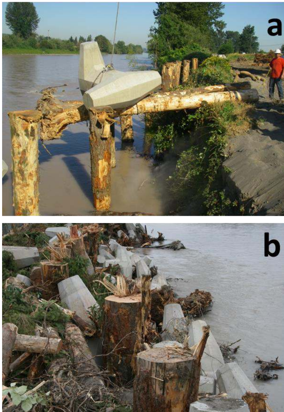
Figure 44A/B. Using a combination of timber and dolosse has been used in Washington State as a more restorative alternative to traditional measures to protect levees and roads. The dolosse are eight ton unreinforced concrete jacks that provide a complex interlocking shape emulating the function of natural snags. The top photo (a) shows how a dolo and attached log can be easily lowered into place and avoid expensive dewatering. Using the dolosse with logs creates a complex structure as shown in bottom photo (b) that can settle if undercut by scour, but without the need of rock or cable. The structures can be designed with lots of wood so the dolosse aren't even visible. Since they are self-settling, these structures don't need to be deeply excavated into the river bed as rock revetments or ELJs constructed only using timber (Figure 42, 43). Photos are of complex revetment built to protect a levee along the Lower Puyallup River in Fife, WA.
