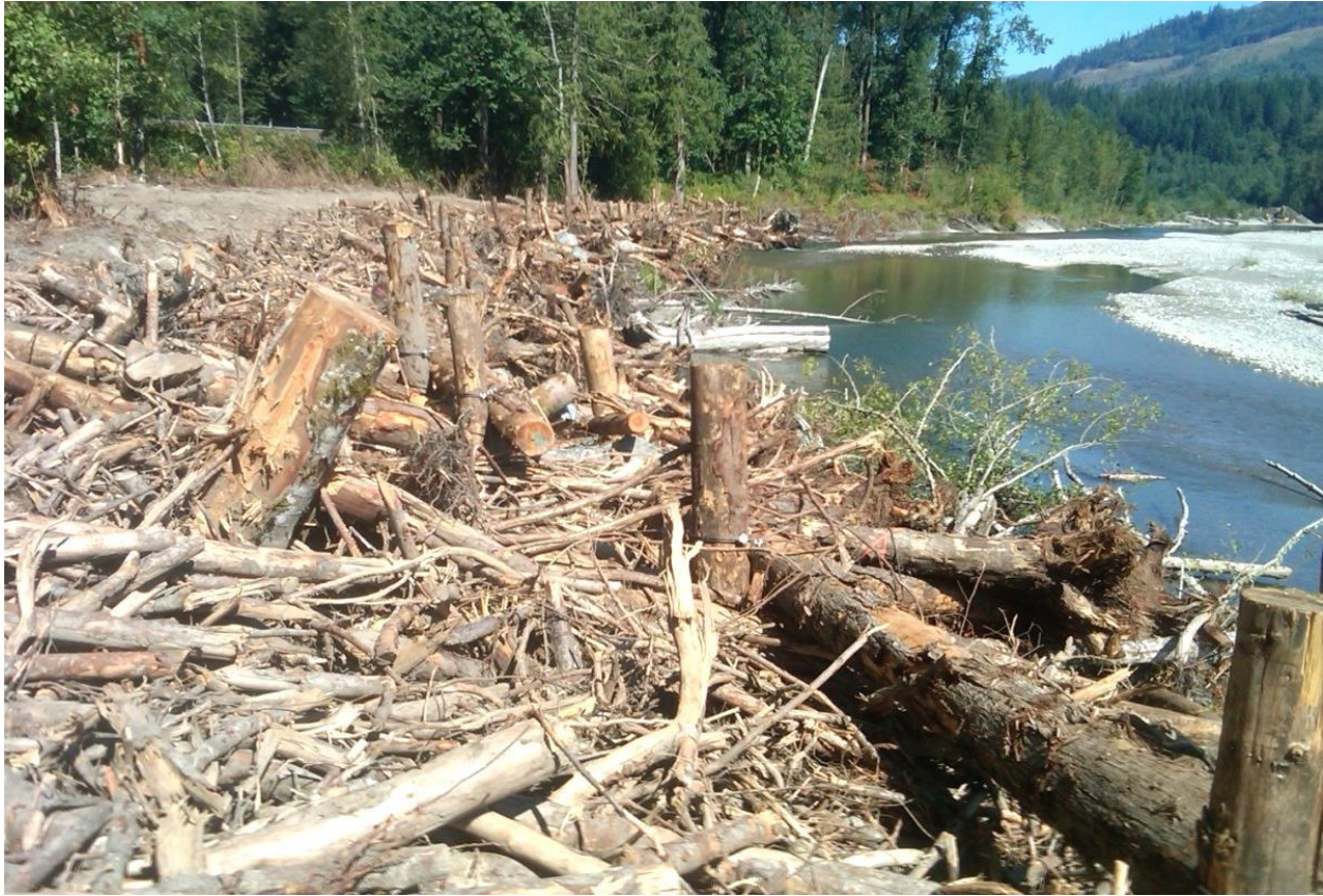
Figure 46. Example of an engineered complex timber revetment bank protection creating a rough shoreline very different than traditional rock revetments found along Sandy River. The structure along the South Fork Nooksack River in northwest Washington is stabilized with timber piles and rock collars (no dolosse). Structure was built in 2011 by Lummi Indian Nation.
