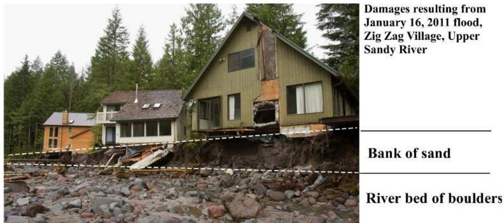
Figure 30. Home damage along the Upper Sandy River due to erosion in 2011 along right bank at Zigzag Village development, RM 45.1. Like much of Upper Sandy, the bank is composed of fine sediment that is more easily eroded than the coarse material of the river bed. Photo credit: The Oregonian newspaper.
