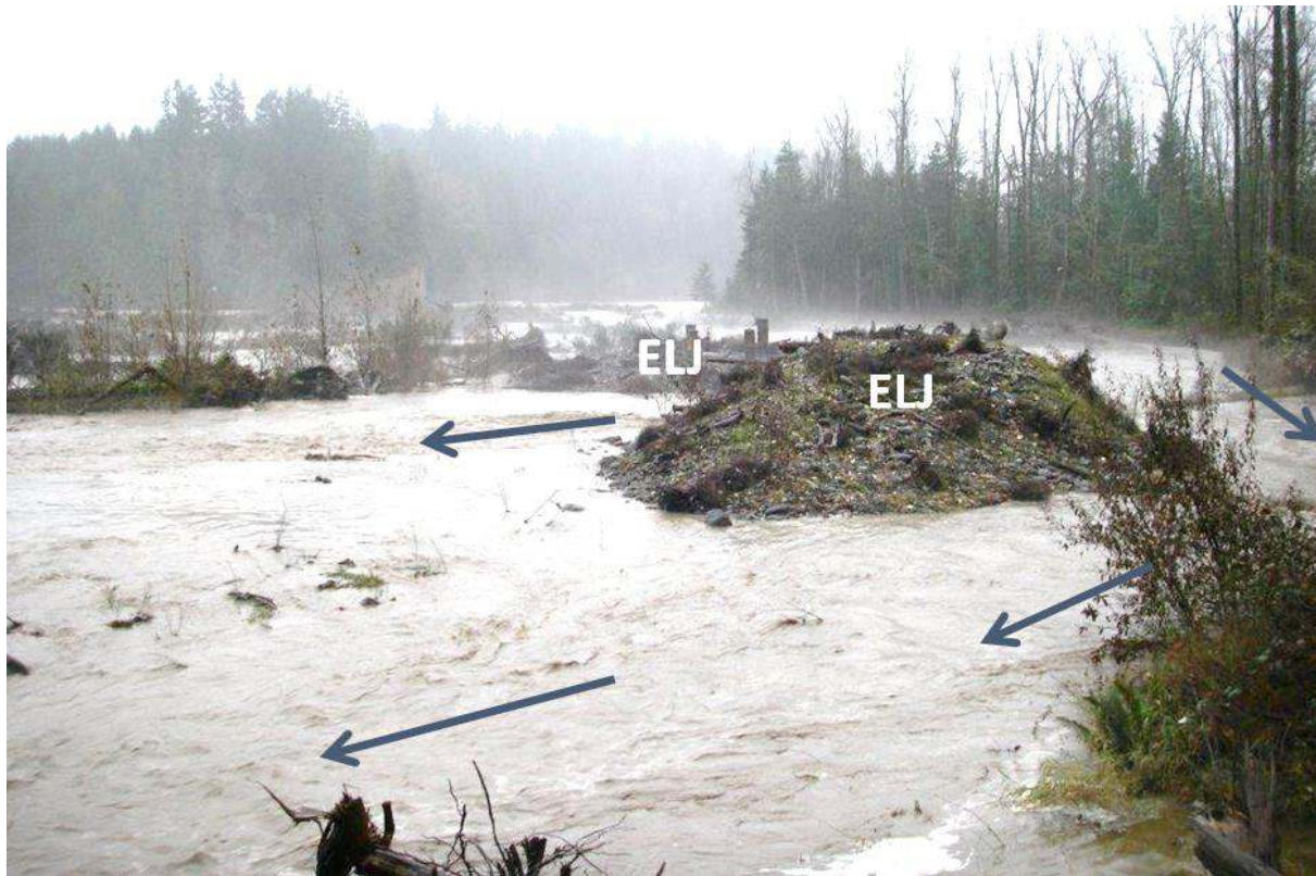
Figure 42. The Upper Puyallup project during high flow in 2014 looking upstream at two of engineered logjams (ELJs) in the energy dissipation area (side channel zone). View is from complex timber revetment on Upper Puyallup River's left bank. The ELJs are splitting flow into smaller channels before the flow reaches the bank. The ELJ is one of six forming an array of structures to keep the main channel from approaching the bank. Photo by Tom Nelson.
