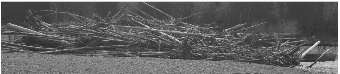
Figure 4. Wood accumulation on a constructed logjam in the Hoh River in 2008, 4 years after construction. Person in foreground gives scale of logjam. The ELJ has accumulated several thousand of pieces of debris ranging in length from 1 to over 20 m and diameters from 0.1 to 1 m. The logjam increases the surface of cover and organic substrate by over 100,000-fold.
