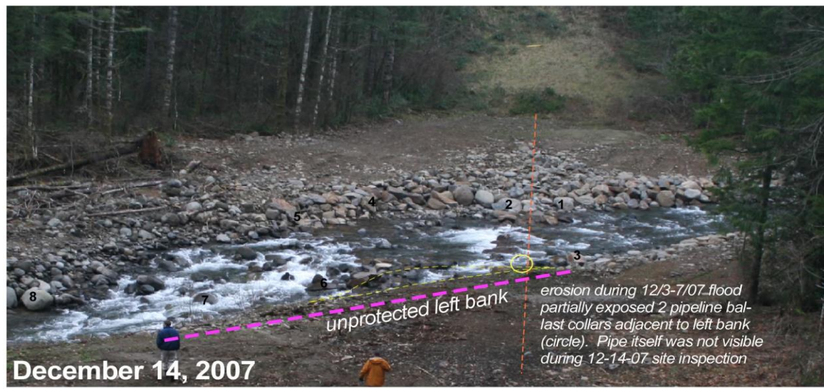
Figure 3. Project site in October 2007 after construction of rock weir (right center) and boulder riffle (left). Boulder riffle was built to raise creek bed so rock weir would not create fish barrier. Site less than 3 months later showed major deformation of boulder riffle, exposure of rock weir and erosion of left bank threatening to circumvent weir.
