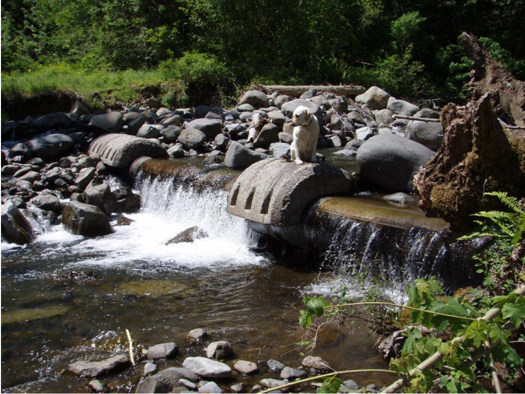
Figure 2. Exposure of pipeline in summer of 2007 after over 2 m of channel incision. Note coarse boulder substrate. Initial treatment was to construct large rock weir immediately downstream of pipeline crossing.
