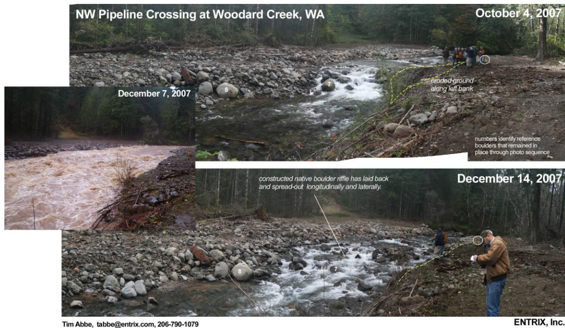
Figure 4. Post construction view looking upstream and again after peak flow on December 7, 2007 (approximately a 1 yr recurrence event, inset photo). December 14 photo shows channel width over boulder riffle almost doubled, eroding into left bank (on right of photo), threatening to cut around weir and re-expose pipeline. Boulder riffle has also laid back its slope and resulted in more exposure of rock weir.
