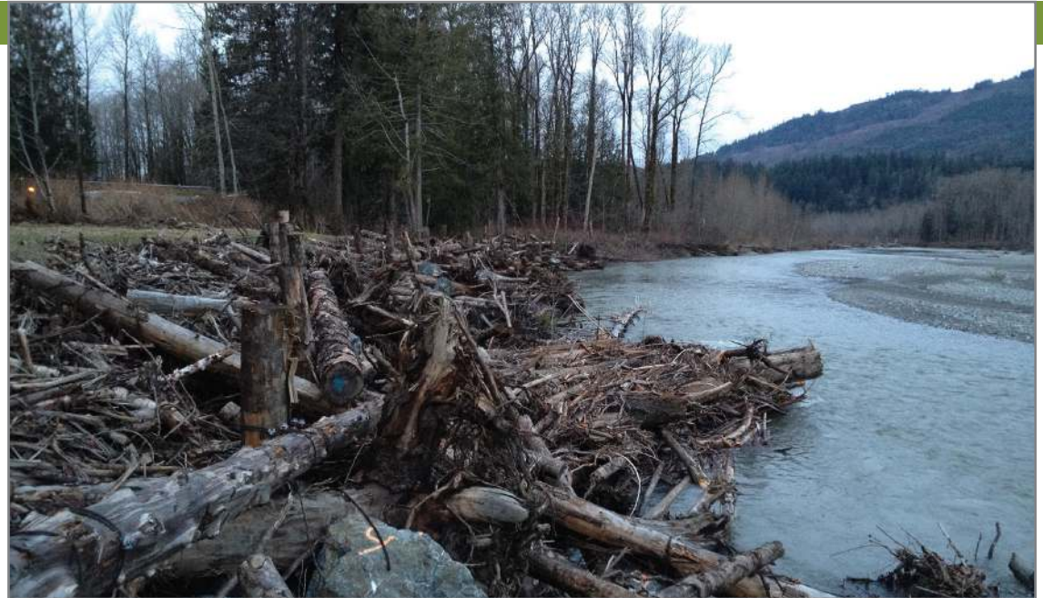
Figure 21. An engineered large wood revetment built by the Lummi Nation created a rough streambank very different than traditional rock revetments found along Sandy River. The structure along the South Fork Nooksack River in northwest Washington is stabilized with timber piles and rock collars. Photo: T. Abbe
