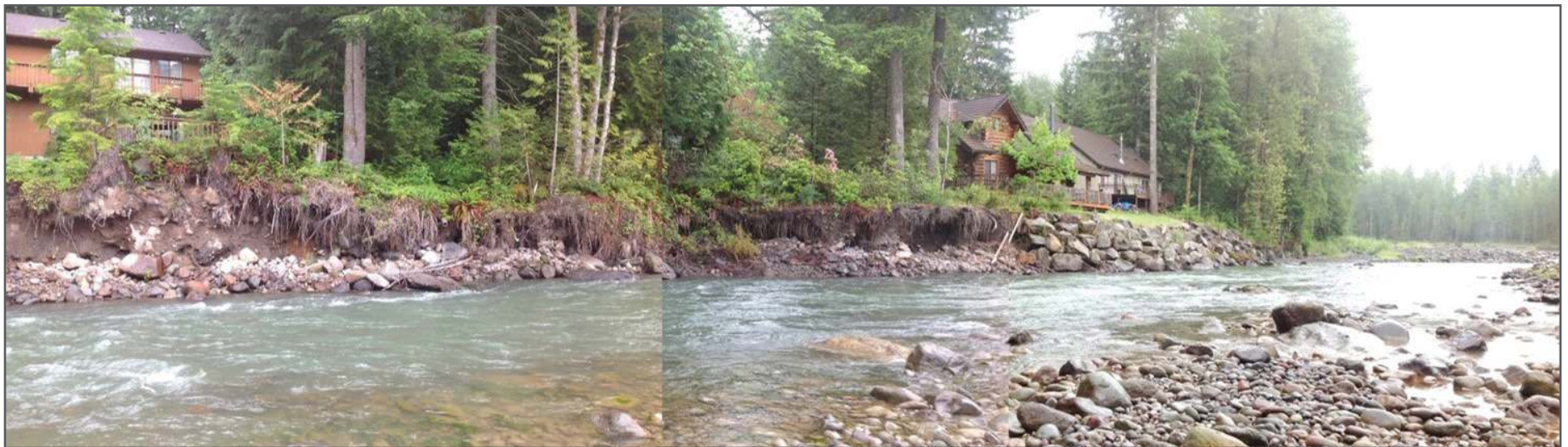
Figure 14. Tree roots can help stabilize banks by adding cohesion, but only to depths of about three feet and thus can be undercut along high banks. A traditional rock revetment (Sandy RM 39.5) is visible in the right background. The relatively smooth surface of these types of traditional bank stabilization structures can intensify erosive energy along natural banks, creating a condition where the structure can accelerate its own demise. Revetments such as this one temporarily slowed river's natural expansion toward its pre-floodplain prior to the Old Maid mudflows. The wider the floodplain, the more the river's erosive power is reduced. Allowing the river space to move and create new floodplain not only reduces flood and erosion risk, but enhances salmon habitat. Photo: T. Abbe
