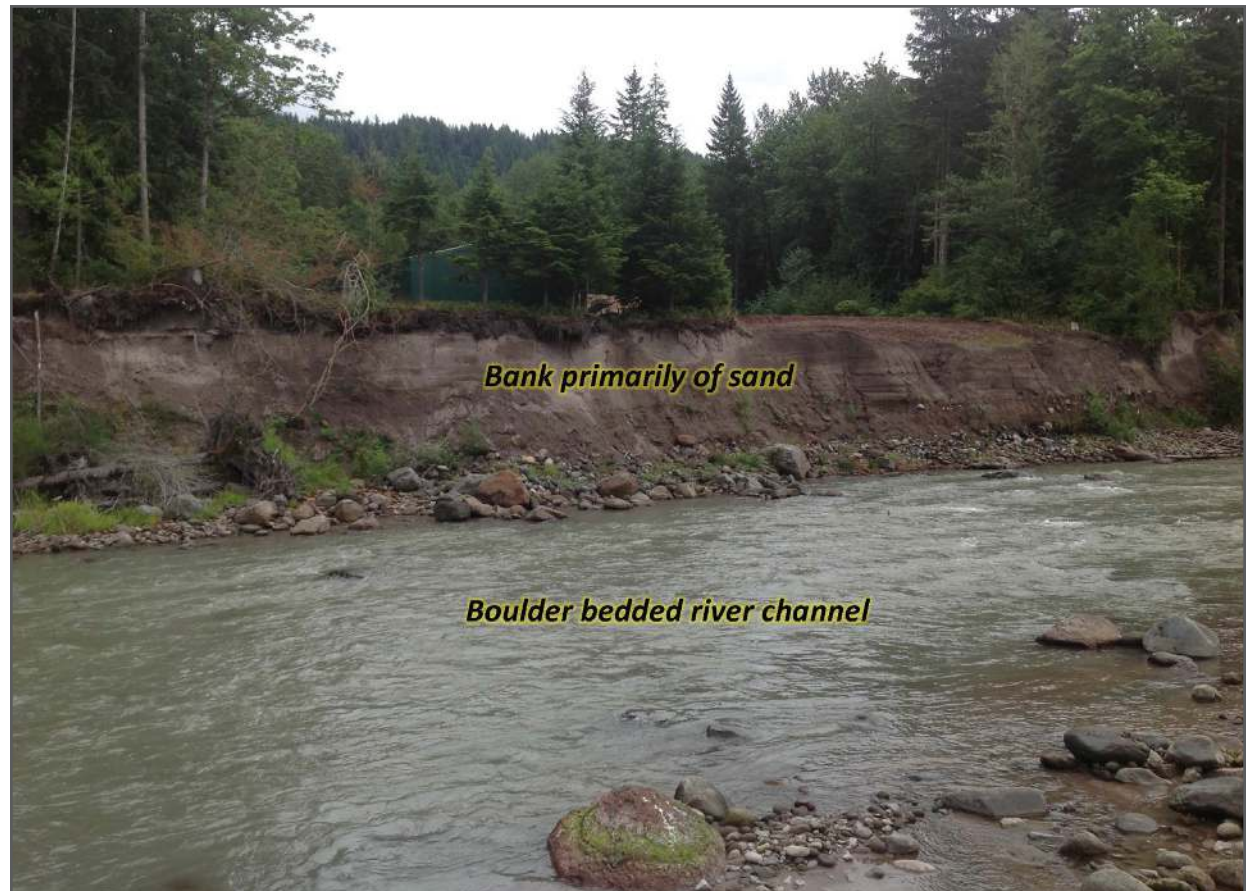
Figure 3. A twenty foot high section of the river's right bank (Sandy RM 40.8) illustrates that homes located well above the zone of flood inundation face serious risks of erosion. The bank is composed of Old Maid mudflow deposits from the 1800s, consisting primarily of sand easily eroded by the Sandy River. Photo: T. Abbe
