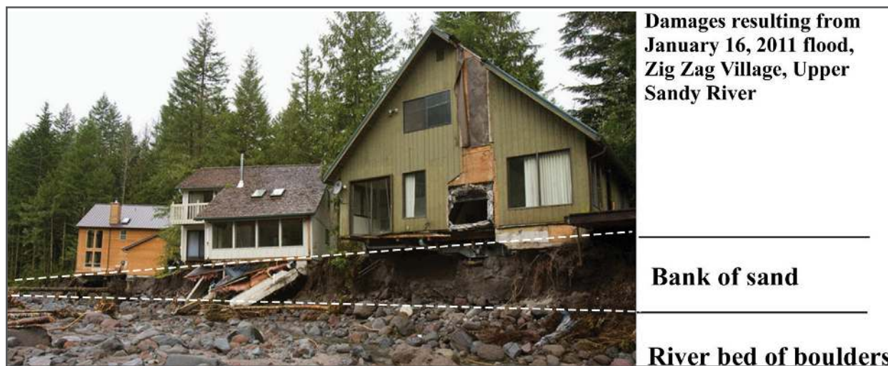
Figure 8. Home damage along the upper Sandy River due to bank erosion. Note the bank is primarily composed of easily erodible sand whereas the river bed consists primarily of boulders. Photo: The Oregonian.
