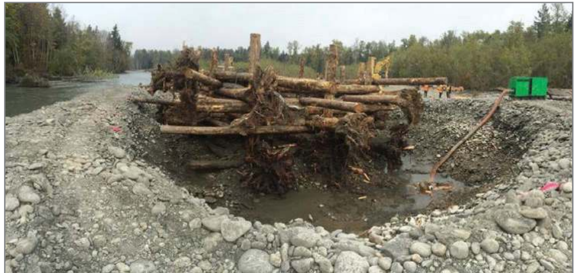
Figure 22. Example of engineered logjam that does not have self-settling elements of previous examples. This structure is deeply embedded into the river so that it can withstand scour without being compromised. Note people on right side of the structure. Pit is 16 feet deep and timber posts extend deeper. Elwha River 2014. Photo: T. Abbe
