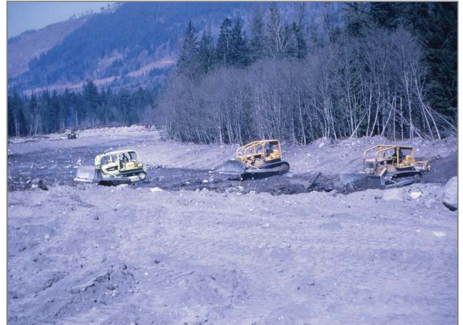
Figure 13. The the U.S. Army Corps of Engineers moved an astounding amount of flood debris in response to the December 1964 flood, here they are re-building the pre-flood channel, confining miles of the Sandy between levees, and stripping off streamside vegetation. Note the fine grained material of sand and gravel. The wide expansion of the river channel and its floodplain that occurred in the 1964 flood left behind large deposits of fine grained material not found in segments of the river that are constrained. The finer substrate not only reflects a less erosive river, but is much more beneficial to salmon. Where the river is allowed to migrate and widen its floodplain, it will create a more sinuous and multi-thread channel that is more effective at dissipating energy and creating more desirable fish and wildlife habitat. Photo: Courtesy of the Arrigotti family and Clackamas County.
