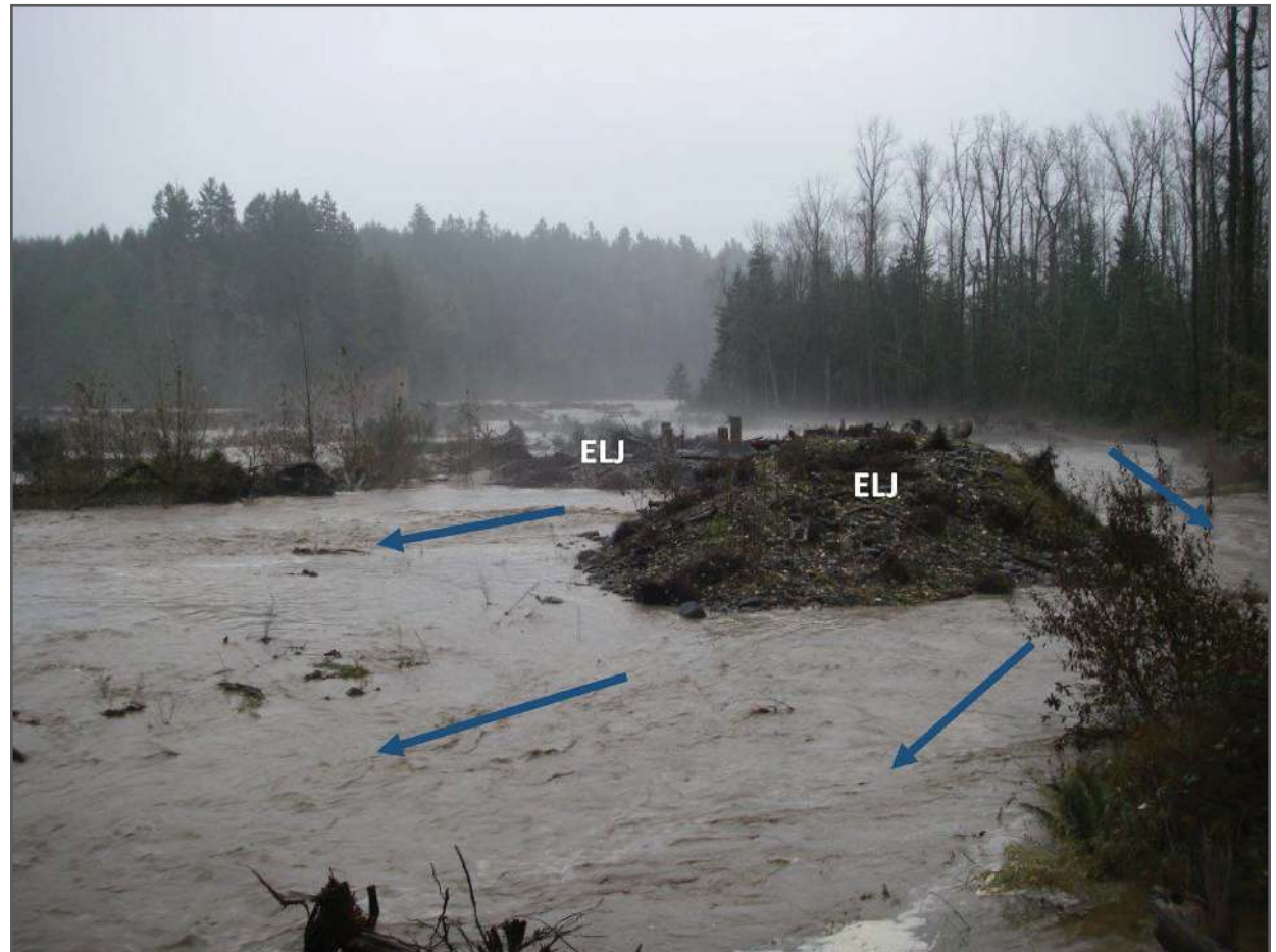
Figure 23. The Upper Puyallup project during high flow in 2014 looking upstream at two of engineered logjams (ELJs) in the energy dissipation area (side channel zone). View is from complex large wood revetment on Upper Puyallup River's left bank. The ELJs are splitting flow into smaller channels before the flow reaches the bank. The ELJ is one of six forming an array of structures to keep the main channel from approaching the bank. Photo: Tom Nelson, Pierce County Public Works.
