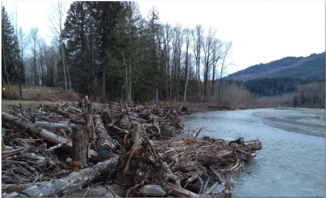
Complex timber revetment designed to protect bank by partitioning shear stress while also creating cover and hydraulic refugia for salmonids, South Fork Nooksack River, Northwest Washington (Tim Abbe 2012)
