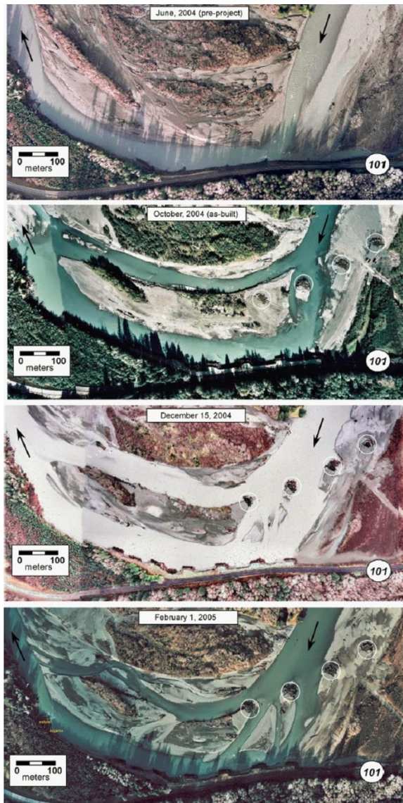
Figure 6-8. Example of the Use of Two Sets of ELJs in Bank Protection Along Hoh River
