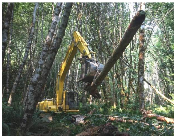
(a) Use of excavator with bucket and hydraulic thumb to position log with rootwad. (b) Use of rotating grapple to move multiple small logs. (c) Log tongs used to position rootwad log in tight quarters.
