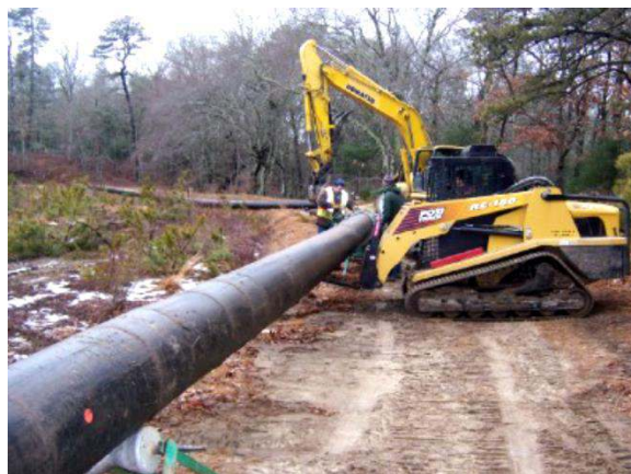
Figure 8-3. Diversion of a Small Stream Around a Construction Zone Through Plastic Pipe
