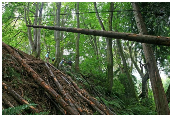
Figure 8-11. Cable Yarding Large Wood for Transport to Channel
