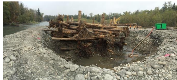
Figure 2-7. Excavation and Dewatering During Construction of an Engineered Logjam in Elwha River, Washington
