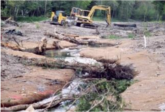
Photo i. Headwater or small perennial stream construction can use wood scaled appropriately to provide overhead cover and bank stability that can last 100 years or more (Photo by Inter-Fluve).
