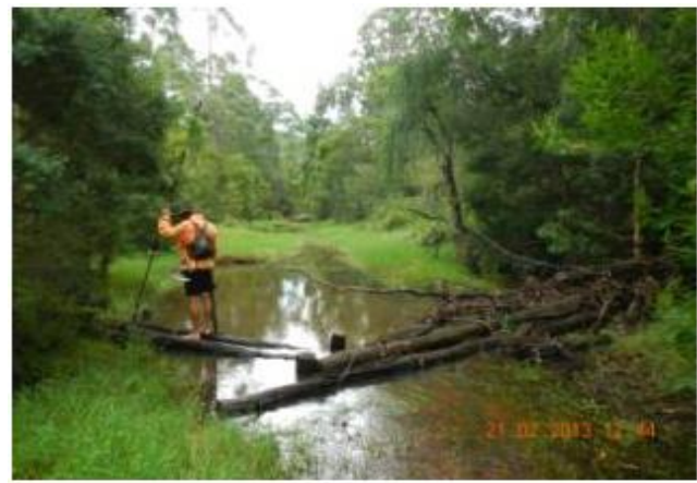
Photo b. Constructed bed control large wood structure in Australia (Andrew Brooks).
