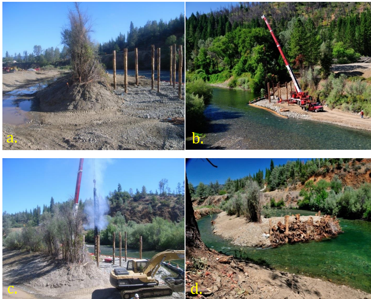
Figure 8-12. Sequence for Constructing Large Wood Structure With Vertically Driven Piles Used to Secure the Structure
