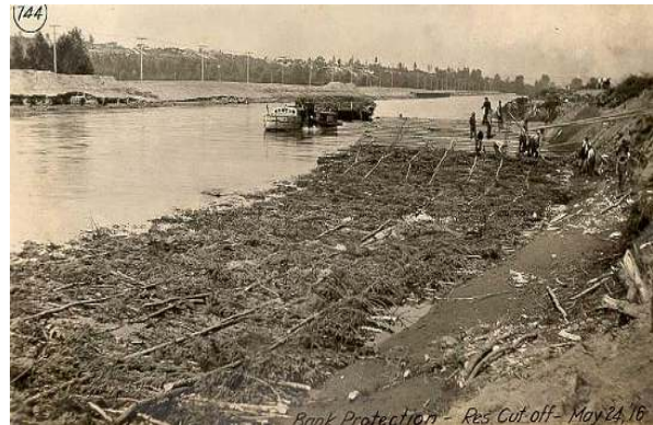
Photo b. Placement of cedar brush mattress along toe of Puyallup River North Levee, May 24, 1916 (photo courtesy of Pierce County, Washington).
