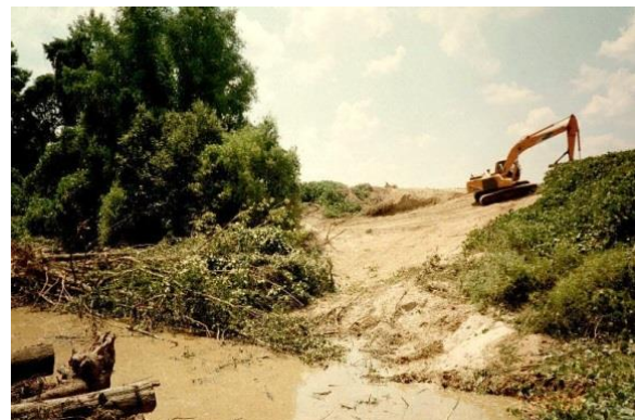
Figure 6-16. Construction of Temporary Ramp for Access to Channel for Large Wood Structure Construction in Little Topashaw Creek, Mississippi
